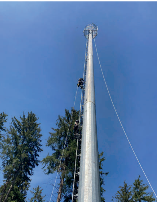
IdentiFlight deployment above the forest canopy on a 40m steel tower.
