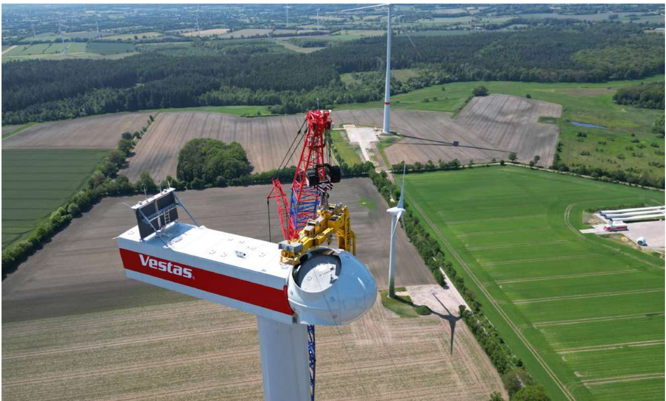
Installation of the scar at the wind farm Reher in June 2023 (Photo J.Weidkamp)
