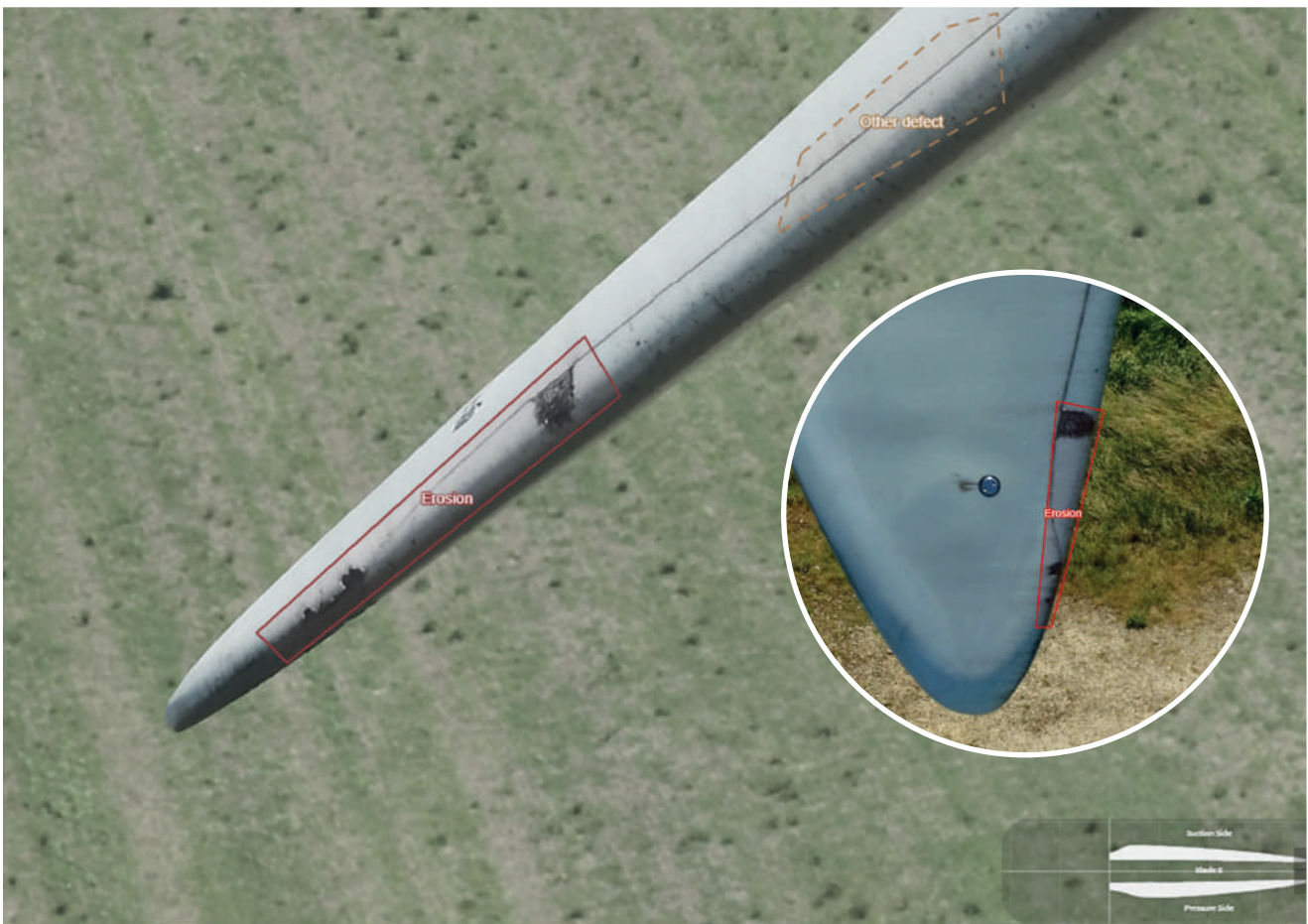
Examples of defects detected in wind turbines.
