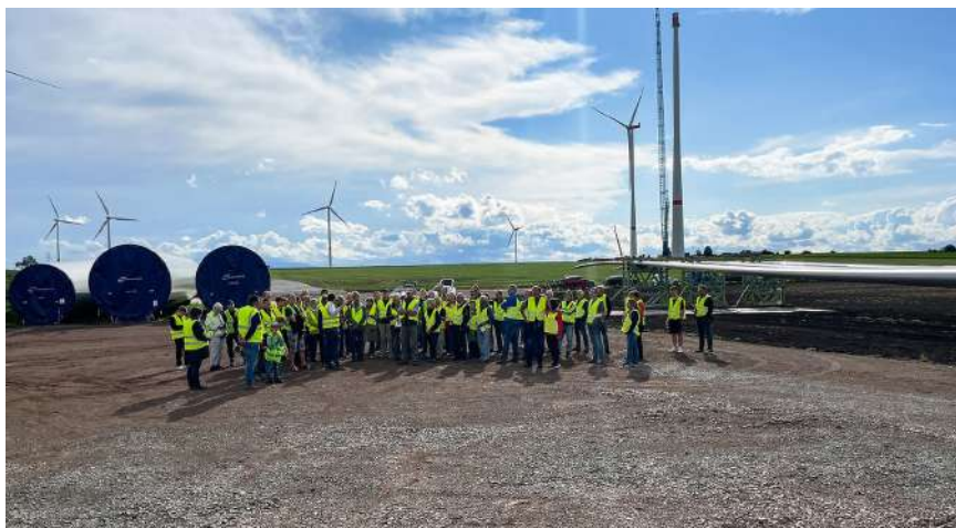
Construction site assembly at Windpark Gevensleben
