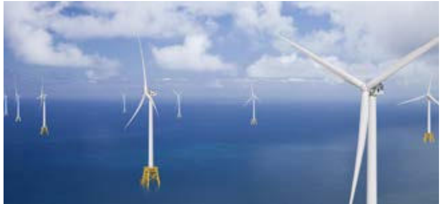
GE's Haliade-X with a 12 MW direct drive generator. Photo: GE
