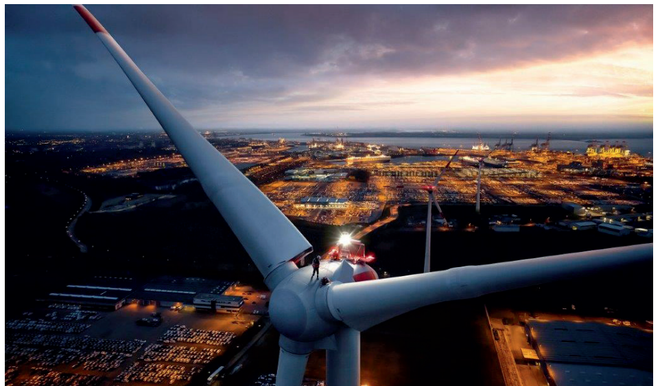
Stunning view: This wind turbine has a hub height of 149 meters and rotorblades with a length of 57 meters.
